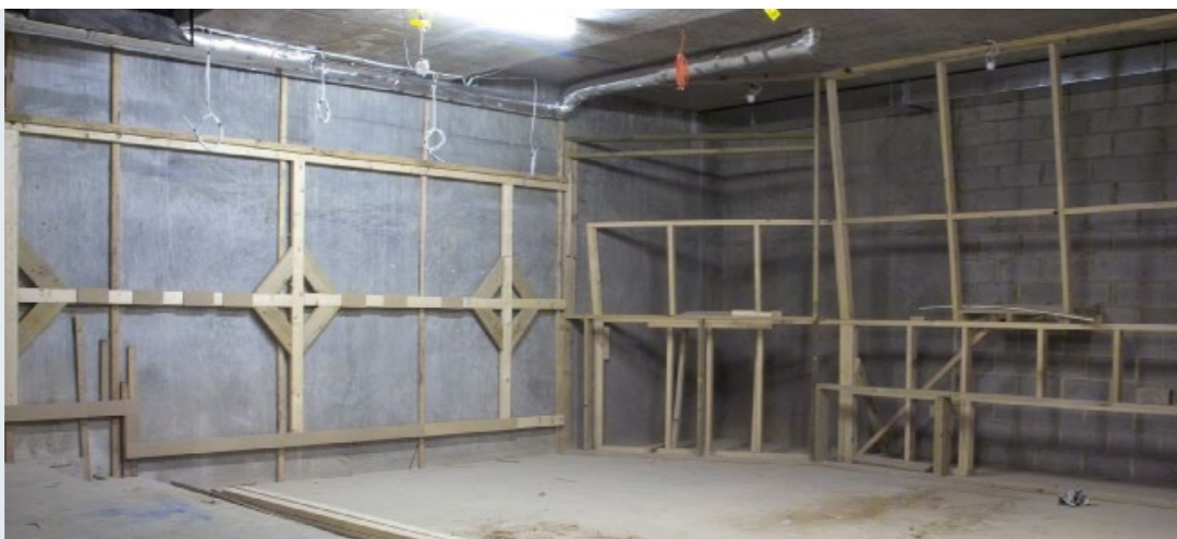
▲ Framing up prior to the installation of equipment and the FabriTRAK acoustical wall system; ▼ Paul Kutcher (left) and Steven Spurrier size up the Genelec speakers behind the 212-inch screen.
